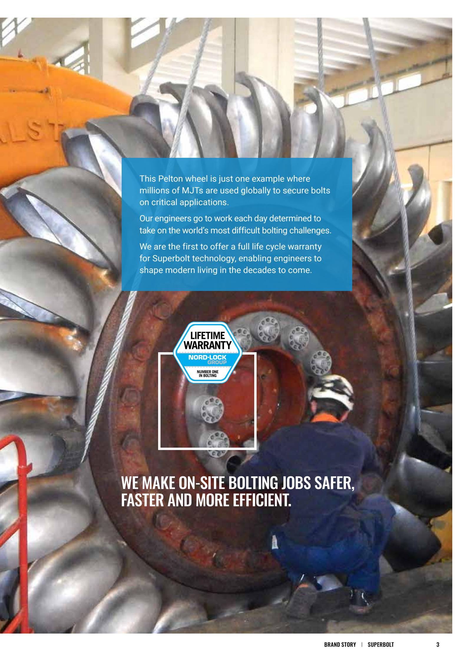
This Pelton wheel is just one example where millions of MJTs are used globally to secure bolts on critical applications.
