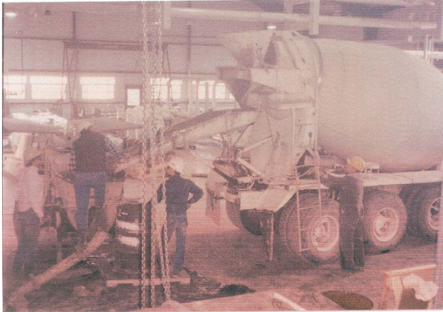
Figure 29 View showing charging of the concrete pump
